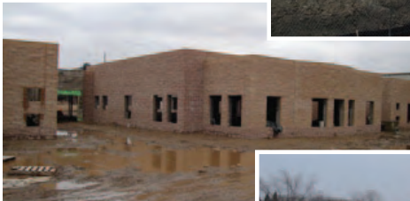
Preschool construction "Hearth and Home"
