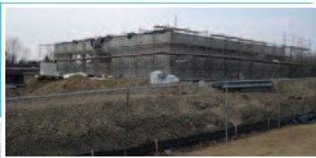
Thurston Multi-Purpose and Preschool classroom construction
