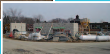
Allen Preschool room construction
